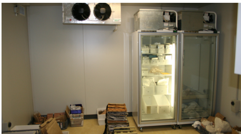
Figure 4: Tasmanian Seed Conservation Centre, Australia - dry room with sorption dryer unit and -20°C chiller cabinets for seed storage.
